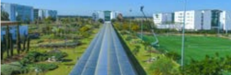
CASANEARSHORE OFFSHORE ZONE
